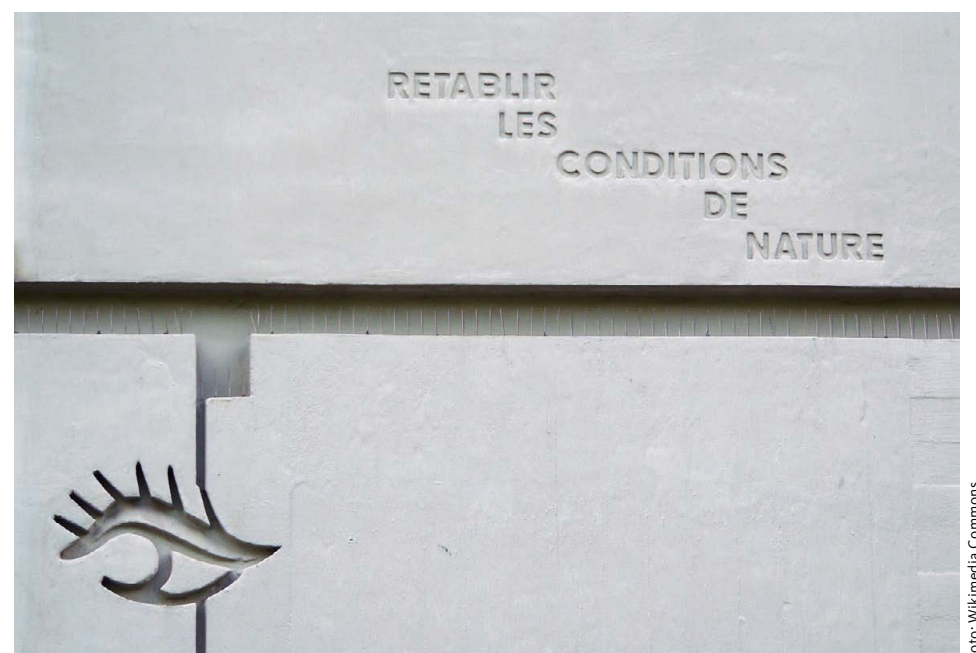
Le Corbusier, Fassadendetail, Unité d' Habitation, Interbau Berlin, 1956–1957
